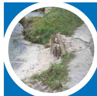
Repaired path and new bank revetment
