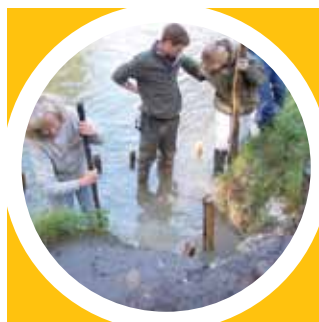
Volunteers install wooden posts
